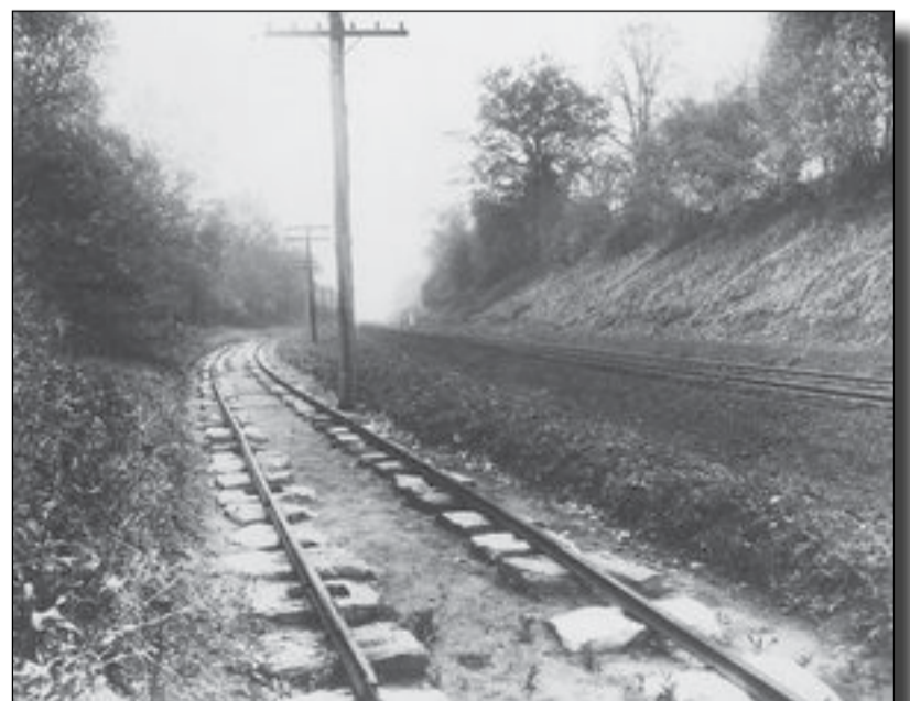
Tracks constructed with "Stone Sleepers"
