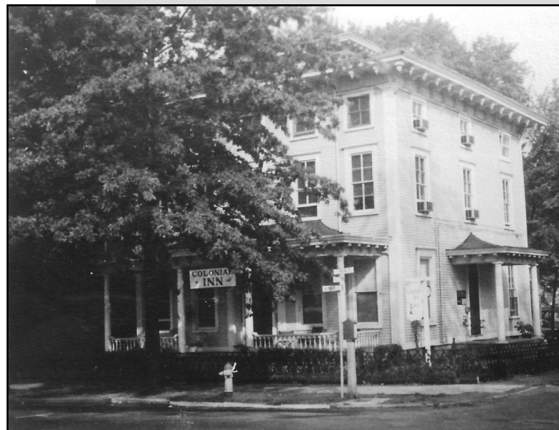
TOP-TO-BOTTOM: Colonial Inn (1 West Main St.), Rulon Hotel, Sumner Residence, Greenleaf (28 E. Main St.)
