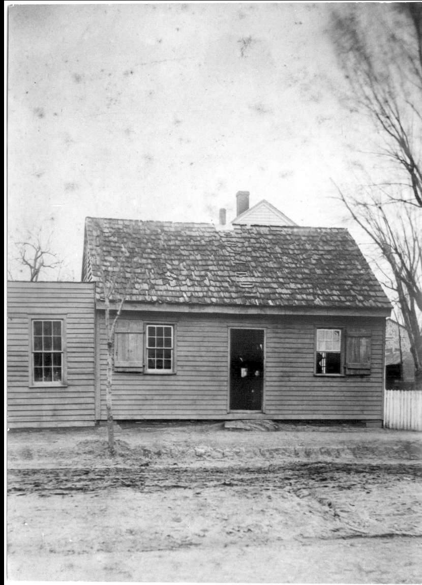
Friendship School at the corner of Church Road and W. Second Street.
