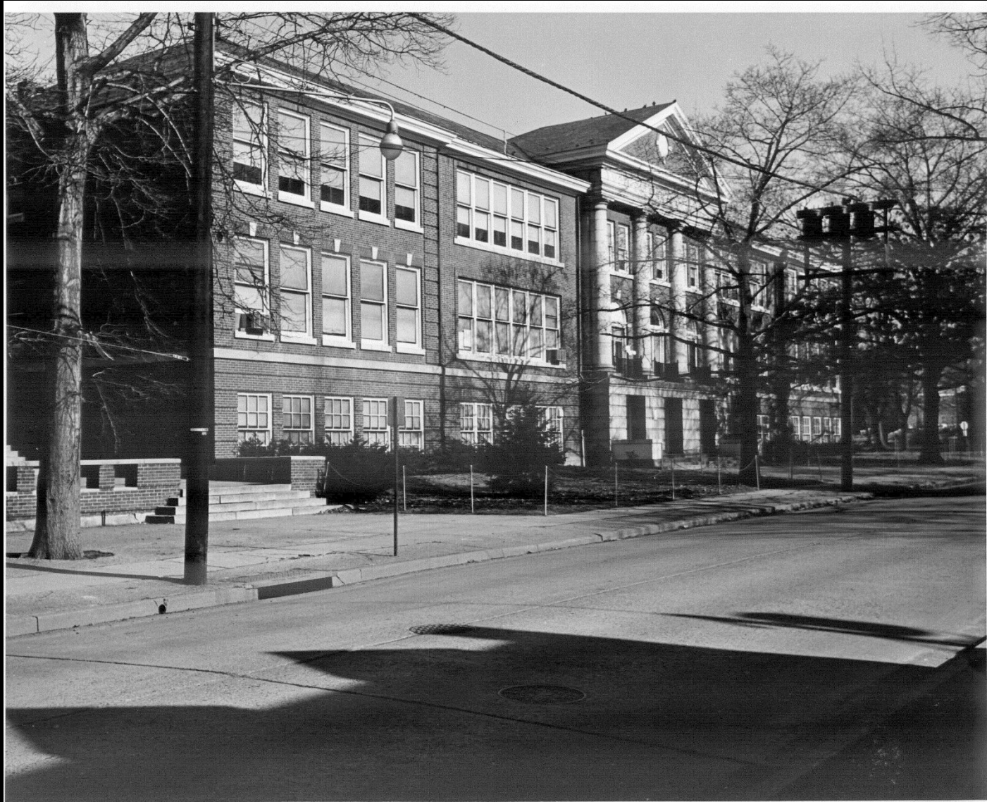
Moorestown High School at the corner of N. Church Street and Second Street
