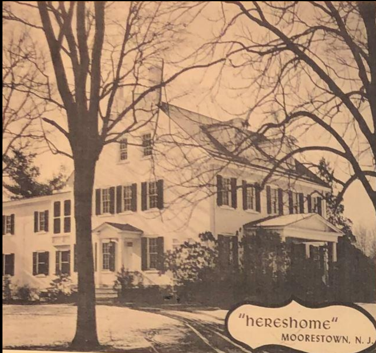
The Home of William Rhoads, "Hereshome", on Riverton Road
