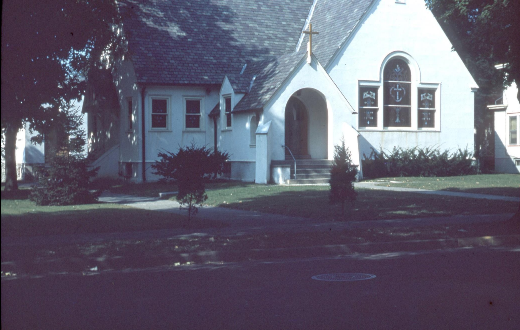
Lutheran Church (formerly Presbyterian) at 310 Chester Avenue – Demolished 1971
